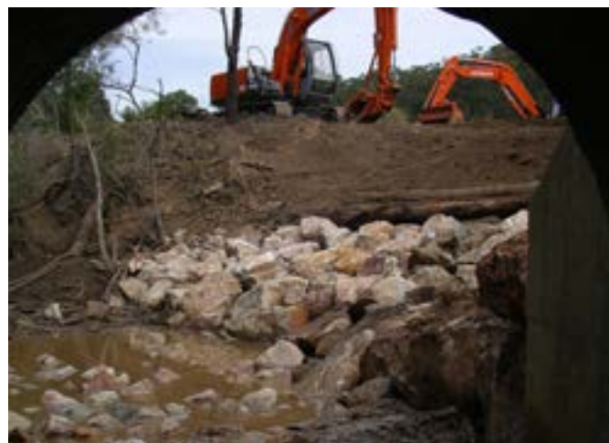
Works at the culvert at Riversdale, near where two creek lines merged into the Shoalhaven River, have involved laying boulders, creating swales for draining, bush regeneration plantings and raising the height of the road. These measures assist in creating a more permanent, stable creek edge which can recover more quickly from flood events. Below flood creek flows at the culvert.
