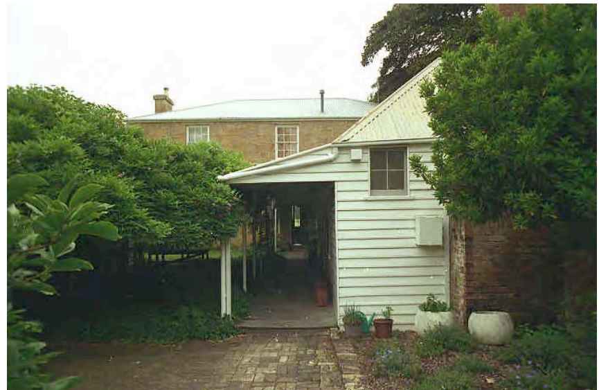
Plate 26 1880's kitchen with external bread oven and flues. Note how the ground levels have risen, obscuring the foundations. Source: Peter Freeman Pty Ltd, 1997
