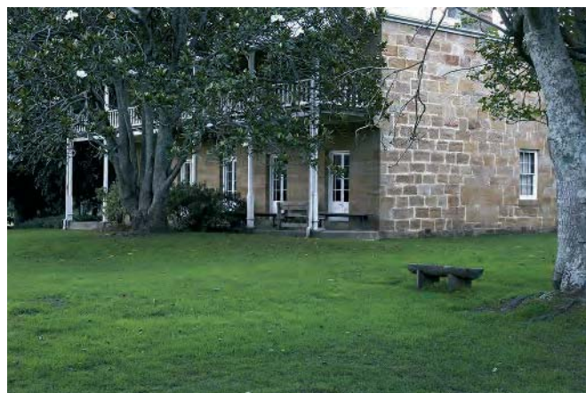
Above: Bundanon Homestead
