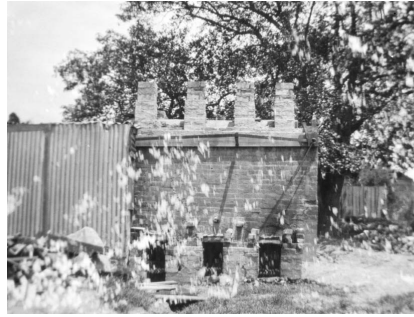
Merric Boyd's eight fire box kiln at Open Country, Murrumbeena, c1917
